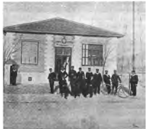
Salonia: The Wireless Station Building.
