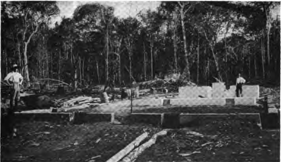
Early Work on the Station.
