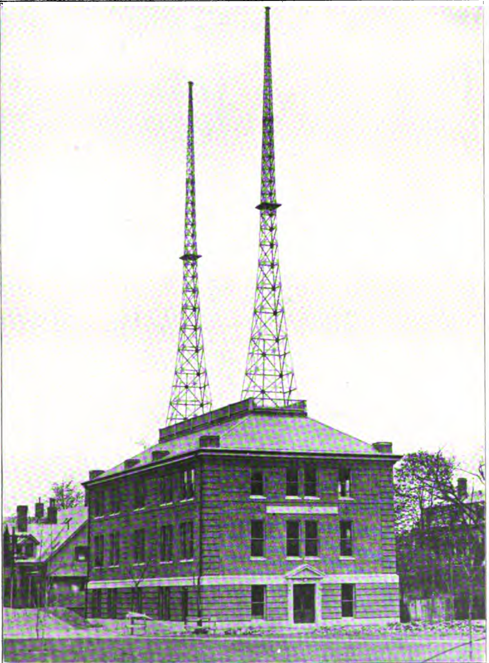
New Croft High Tension Laboratory, showing Steel Wireless Towers.
